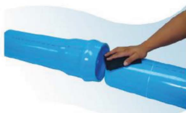
STEP 3 Clean the spigot end of the pipe as far back as the reference line.
